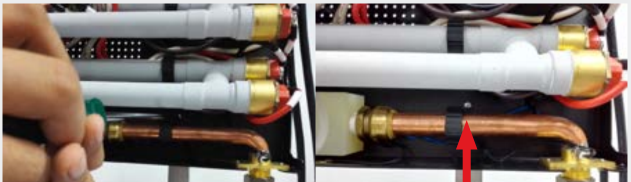
Figure 3. Tightening the Mounting Screws
